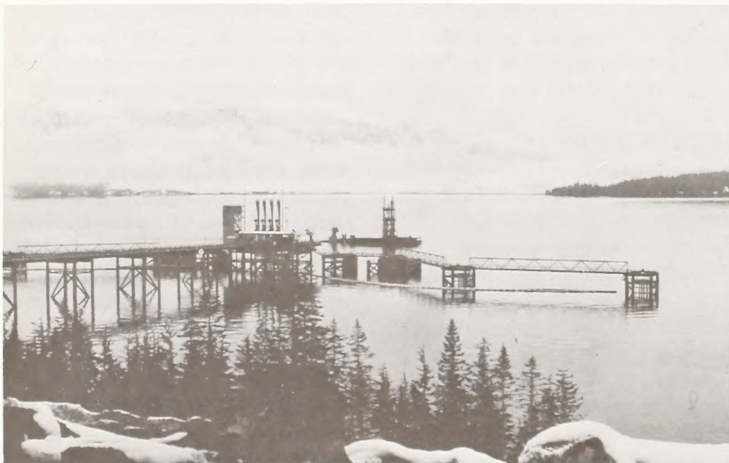
One of the loading berths where Prudhoe Bay crude oil is loaded onto tankers in Valdez Harbor. At this point, tankers pump out their ballast water to be cleansed and later returned to the clear waters of the harbor where the tankers side.
